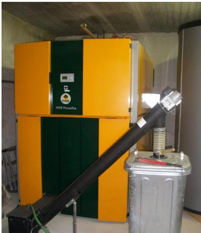
Caldaia a biomassa KWB POWERFIRE TDS 300 kW
